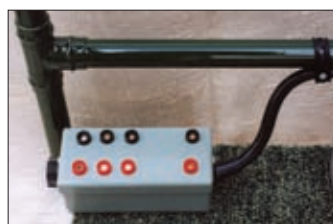
● Fig. 4: The three sets of terminals on the left are the switched and fused supply points, while the single pair on the right make up the charging point for the spill-proof lead-acid battery.
